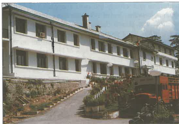
Main building of CPRI at Shimla
